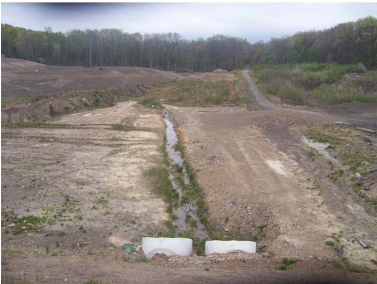
Figure 3. Existing Upstream Section 11 May 2006.
