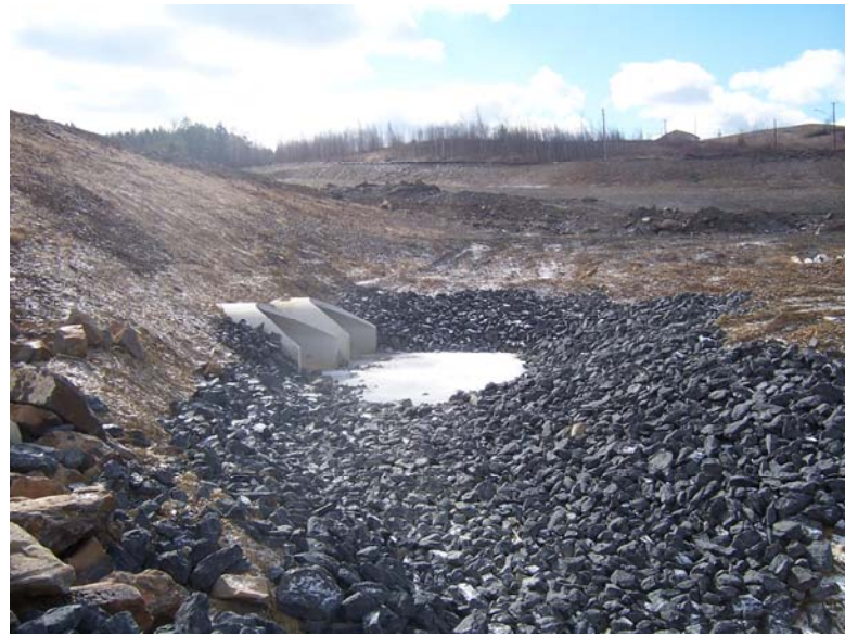
Figure 2. Energy Dissipator 28 February 2006.
