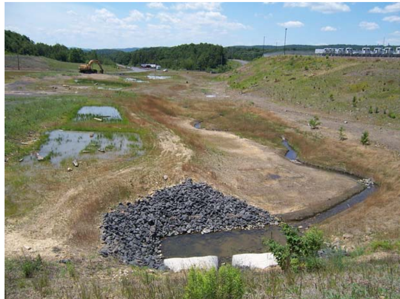
Figure 6. Restored Downstream Section 30 June 2007.
