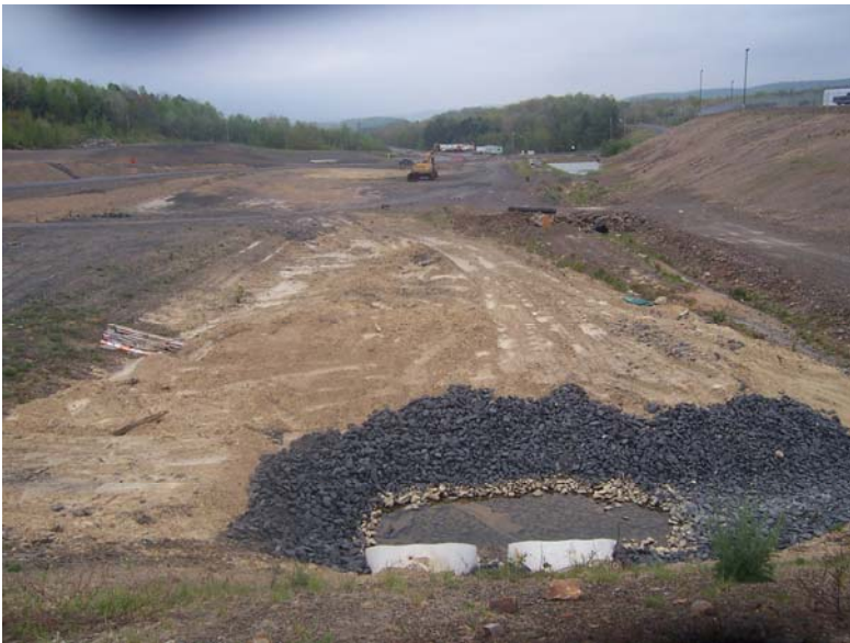
Figure 5. Existing Downstream Section 11 May 2006.
