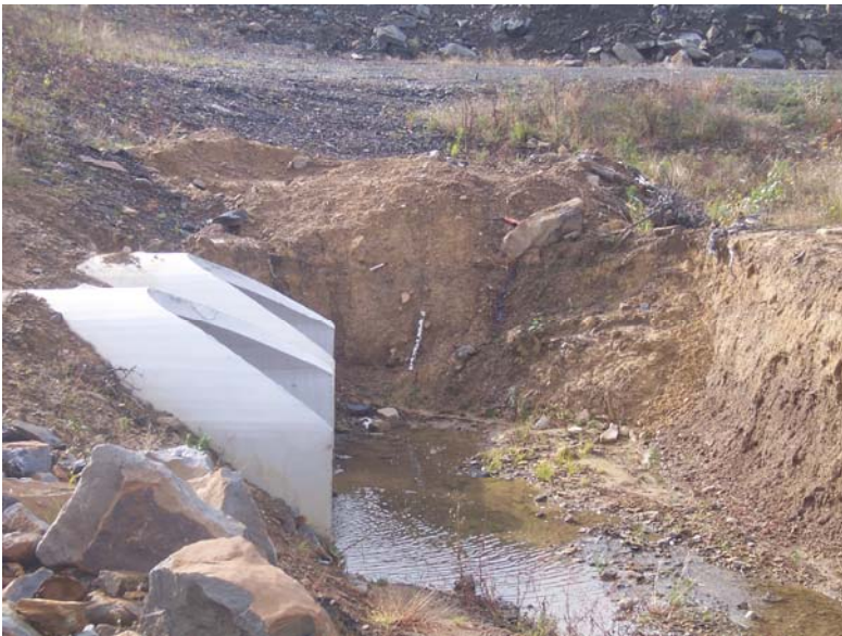
Figure 1. Energy Dissipator 30 November 2005.
